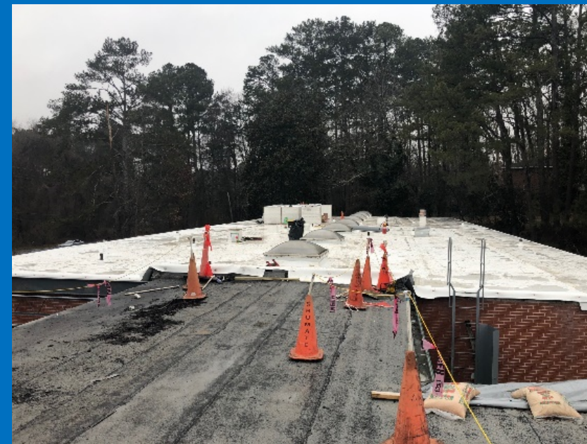
TPO Roofing Replacement
