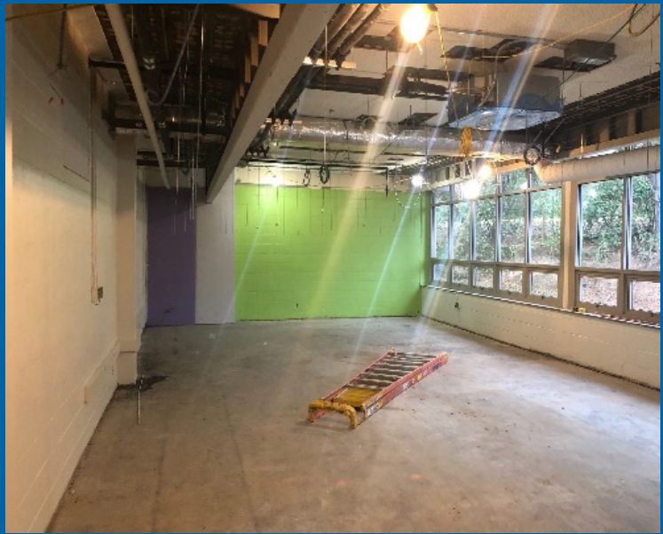
SW Wing Paint and Ceiling Grid Hangers
