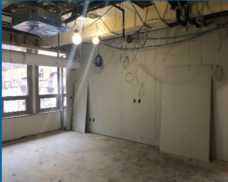
SW Wing Drywall Installation
